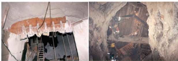
Figure 8—Examples of orepass rehabilitation work
