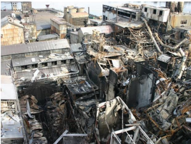
Figure 1—Aftermath of aluminium dust explosion at Hayes Lemmerz International-Huntington foundry<sup>6</sup>
