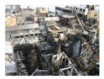
Figure 1—Aftermath of aluminium dust explosion at Hayes Lemmerz International-Huntington foundry<sup>6</sup>
