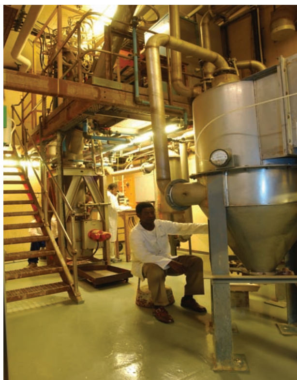
Figure 4—Photo of the plasma-dissociated zircon plant from the ground floor level
