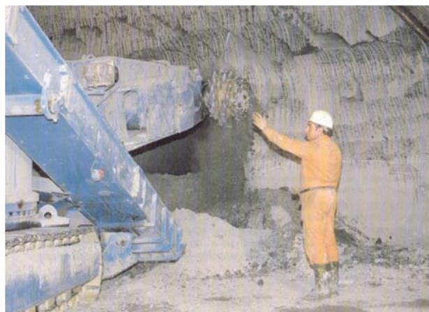
Figure 14—Typical application of GRP bolts where cutter heads are used
