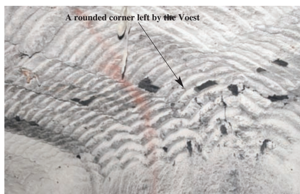
Figure 13—The corner created by the Voest CM showing the scaling that has taken place
