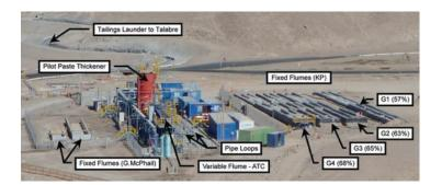
Figure 1-Pilot plant layout
