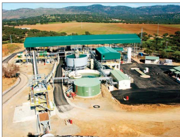
Figure 1b—The Aguablanca treatment plant
