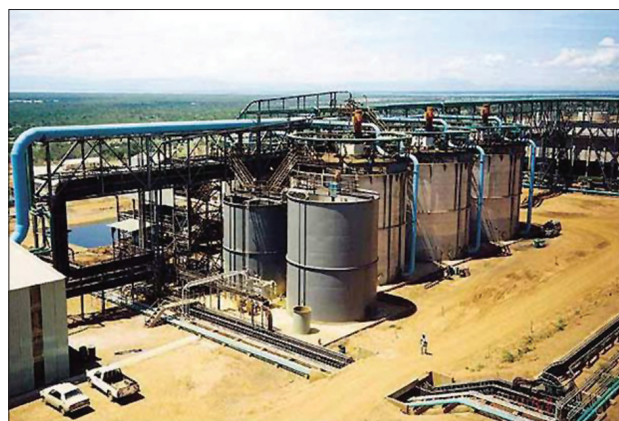
Figure 8—The Kasese bioleach plant, which treats a cobaltiferous pyrite concentrate, comprises six bioreactors each with a volume of 1,400 m 3 . At the time of construction, these were the largest individual reactor volumes for a plant of this type
