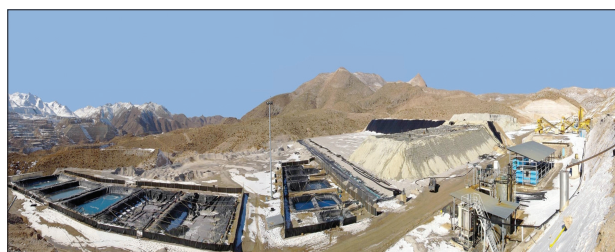
Figure 6—The Mintek-NICICO chalcopyrite copper heap bioleach demonstration plant at the Sarcheshmeh Copper Complex, located in the province of Kerman, Iran
