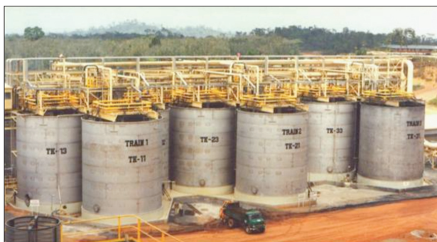
Figure 2 – Bioleach reactors rank amongst the largest high intensity process reaction vessels in the world, as evidenced by these approximately 900 m 3 reactors at the Ashanti BIOX ® plant in Obuasi, Ghana
