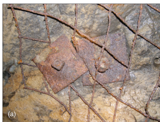
Figure 4—(a) Corroded plates with deteriorating screen; (b) corroded split set ring
