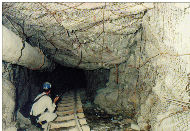
Figure 1—Haulage conditions experienced in the squeezing rock at Hartebeestfontein Mine (courtesy W.D. Ortlepp)
