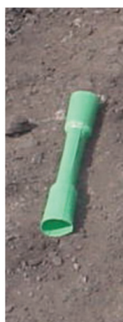
Figure 1—HDPE spacer of 10 cm effective spacing length
