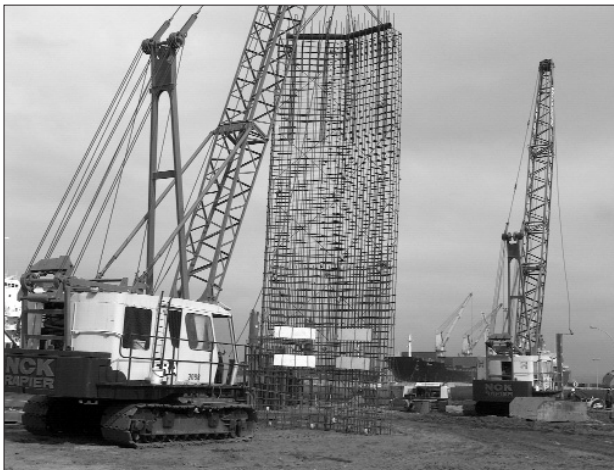
Figure 8—Shaft diaphragm wall reinforcing panel being lifted into position
