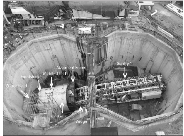
Figure 9—TBM established in the north shaft prior to launch
