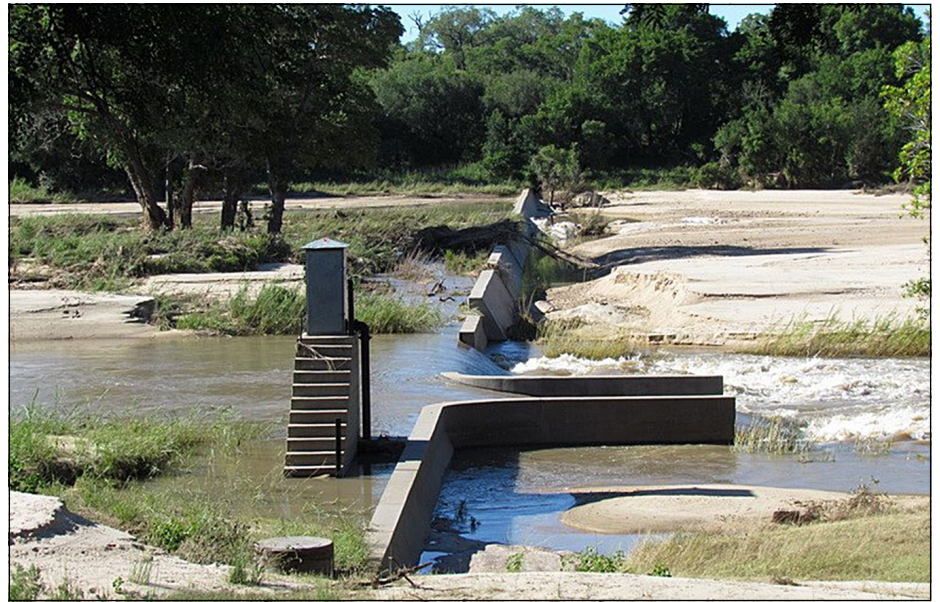
Figure 5 Flow-gauging weir X3H008 in the Sand River (Rademeyer 2023)
