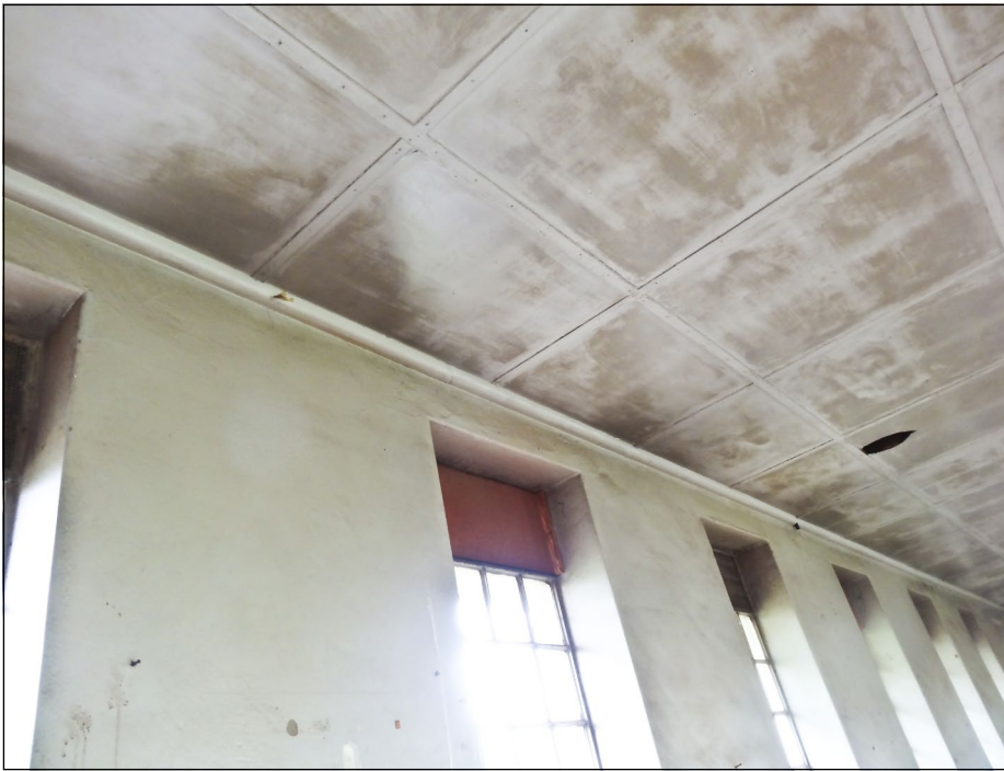
Figure 2 The interior of one of the abandoned buildings illustrating no cracks
