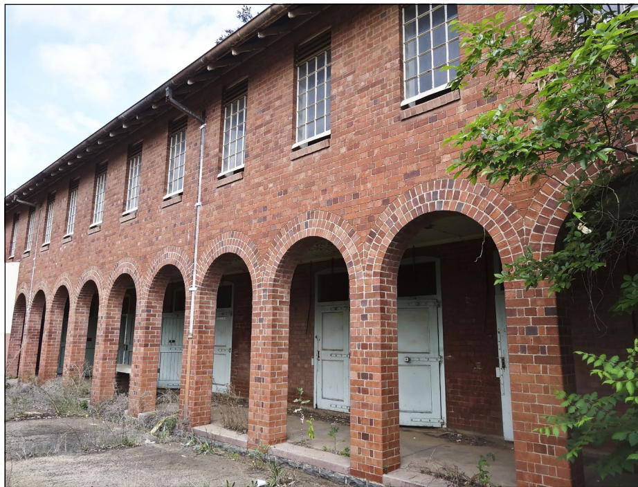
Figure 1 One of the abandoned buildings at the former Oranje Hospital
