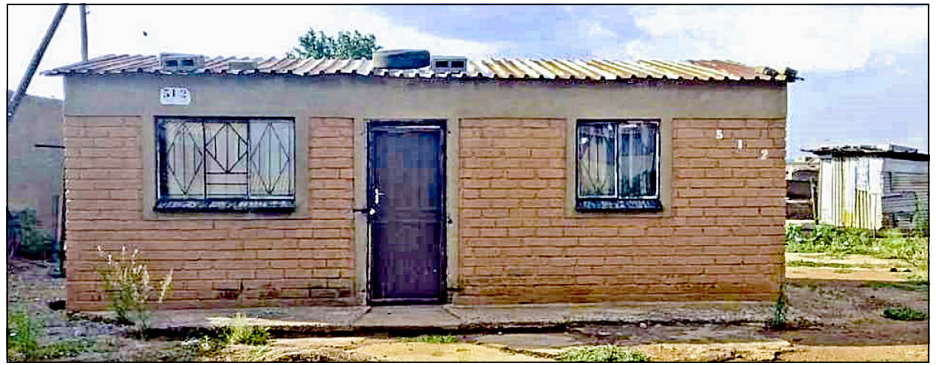
Figure 2 Illustration of heavy objects used to secure a roof of a LIH against wind uplift (Mabuya & Scholes 2020 – photo reproduced here under the Creative Commons Attribution Licence)
