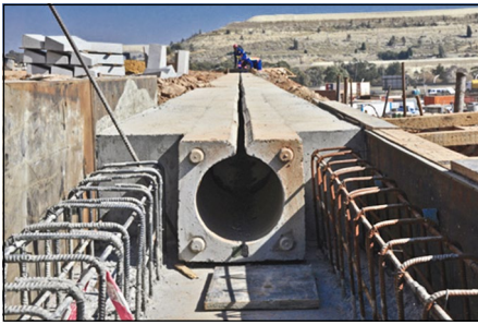
Figure 3 Slotted drain installation
