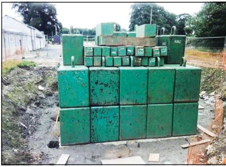
Figure 4 Full-scale load test
