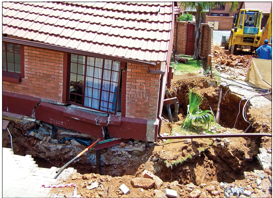
Figure 1 Coincidence of sinkhole with residential house (Centurion, South Africa)
