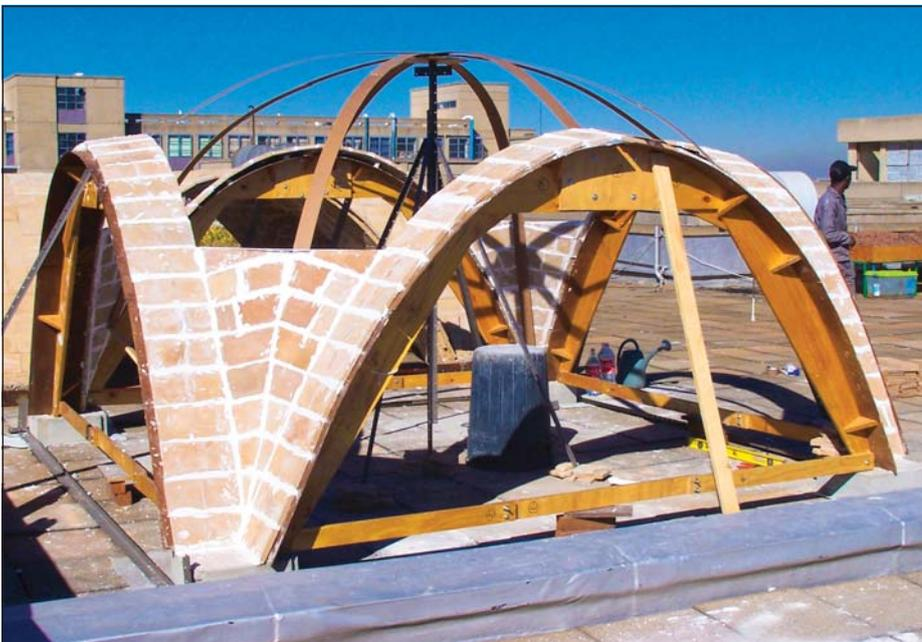
**Figure 12** Masonite strips used as construction guides
