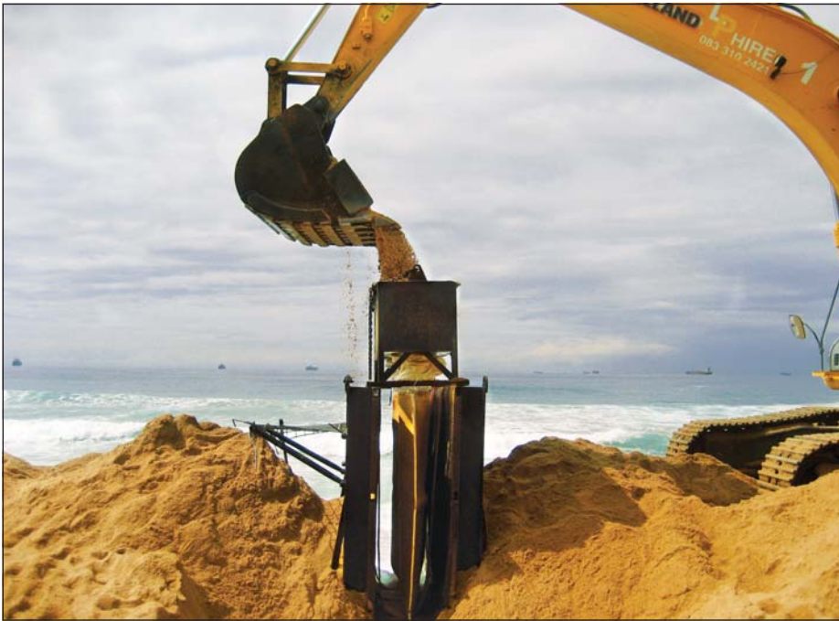
Figure 7 Filling of geotextile sand bags with frame (April 2007)
