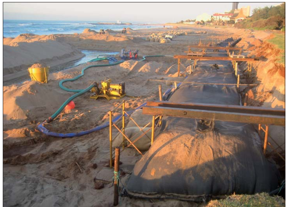
Figure 11 Geotextile tube installation at Amanzimtoti (April 2008)
