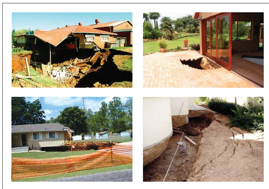
Plate 2 Different scenarios of houses collapsing or hanging over sinkholes
