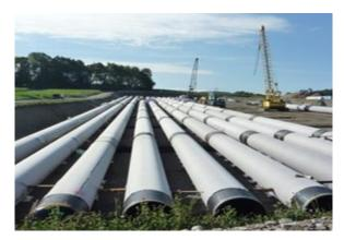
Figure 7: Surface pipeline compressed gas storage (Bilfinger Industrial Services GmbH (BIS), 2021).
