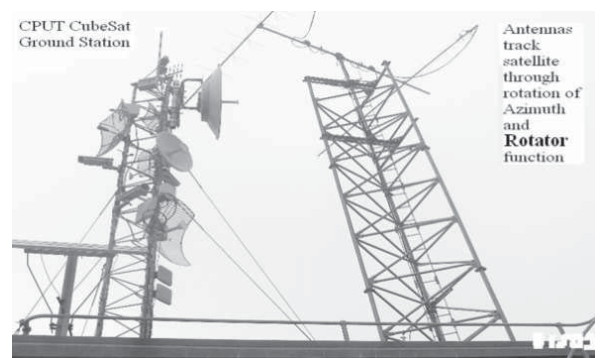
Figure 2: Antennae for satellite tracking
