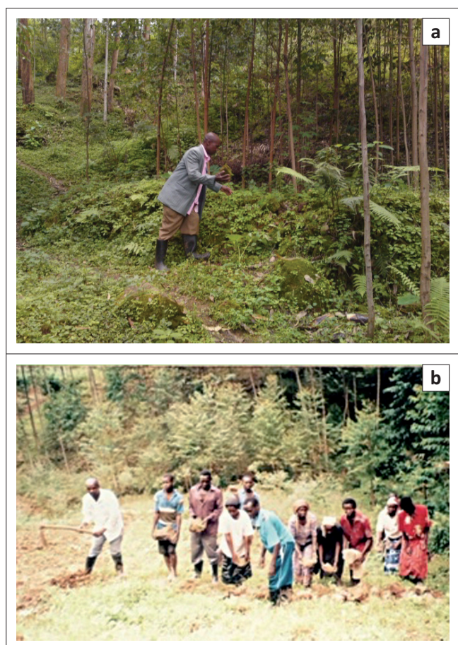
FIGURE 6: (a) Stone terrace (where the person is pointing) and eucalyptus trees planted to stabilise the soils on a scar in Bushika and Bunakasala villages. Note also the underground dense herbaceous growth, which is important for enhanced stability of the soil. (b) The local community members of Shunya Yettana working as a team in digging, collecting and assembling stones along a contour on the landslide scar.
