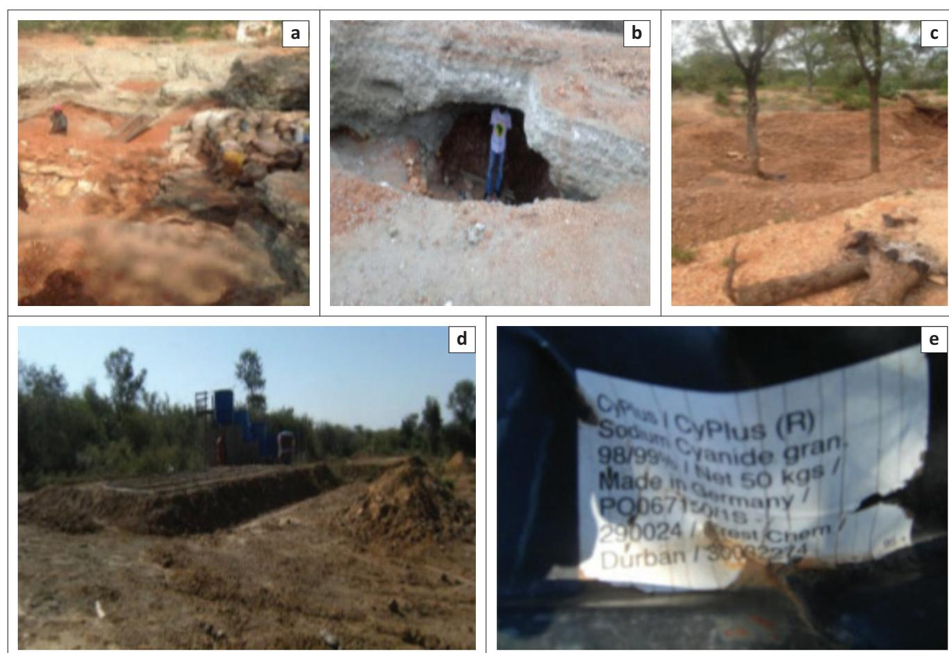
**FIGURE 2:** Artisanal mining at the Sutherland goldfield: (a) Fine gravel digging operations, (b) hazardous excavation at Louis Moore Mine, (c) the impact of excavations on trees around New Union Mine, (d) an abandoned cyanide heap leaching setup (e) and an empty container of the leaching chemical used.
