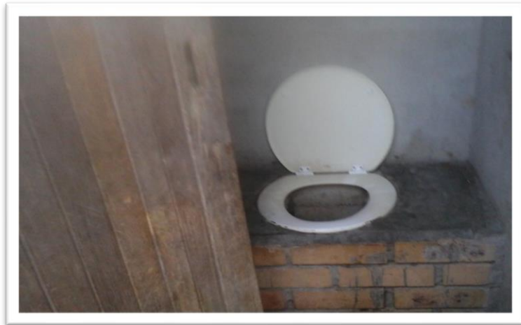
Image 5: Pit Toilet: Tlanga Primary
