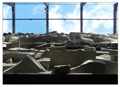
Figure 12: Elevated stacked stone wall acting as a light filter to the interior and the exterior glass wall providing thermal isolation (Auret).
