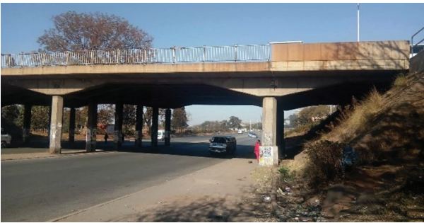
Fig. 12. Partial front view of the Beatrice Bridge
